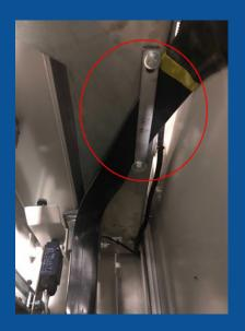
Step 7. Lift the car sling slightly off the ground with the hand crank, and then tighten the bolts
